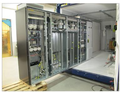
Reassembly of electrical switchboards and container
